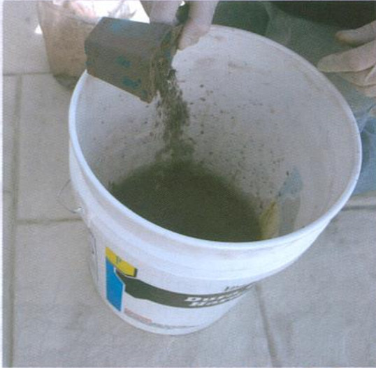
Measure and Mix with Water
